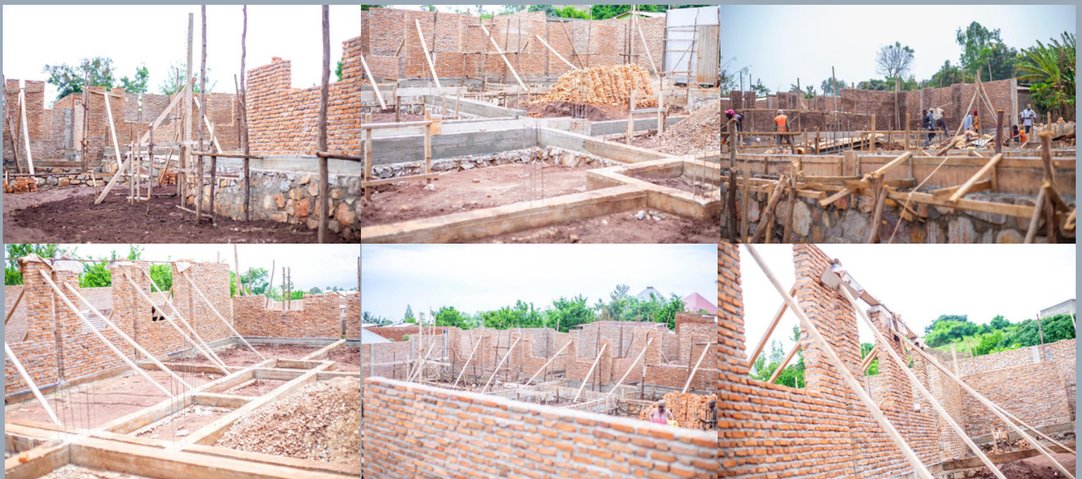
Week 3 and 4: Beginning Masonry
