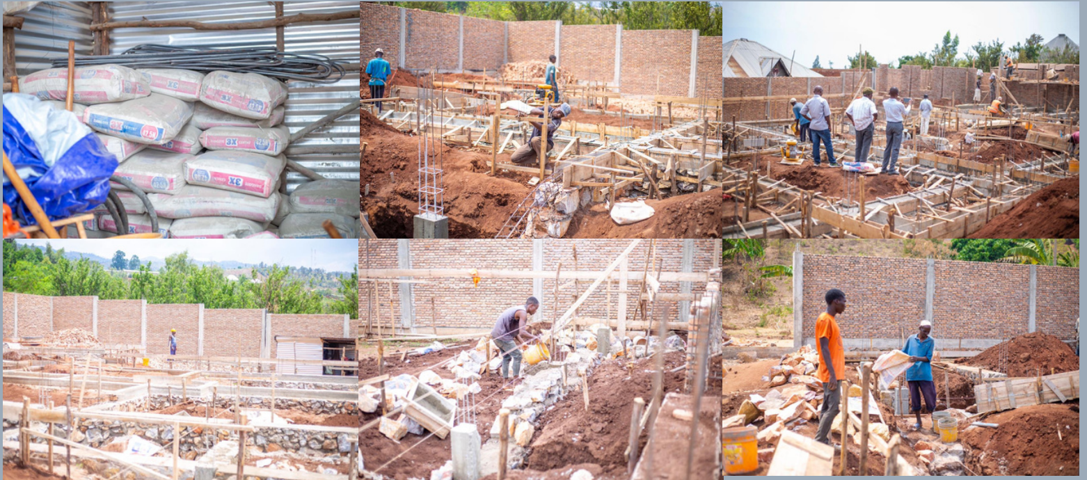
Week 1 and 2: laying the foundation
